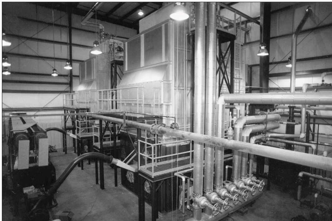
A wood-fired boiler at Kincaid Furniture. Photo provided by Industrial Boiler & Mechanical Co., Chattanooga, Tenn.
