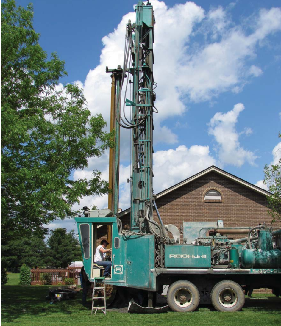
LEFT: A “closed” loop was installed in our yard, which required three 200-foot holes to be bored vertically. The loop field is connected at one central point, passed through our foundation and connected to the unit in our crawlspace. Photo by Cindy Schafer
